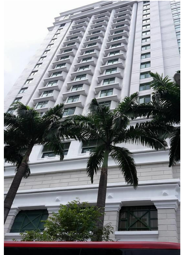
Plaster Walls (Façade Repairs & Granitic Coatings) Ritz Carlton Hotel, KL
